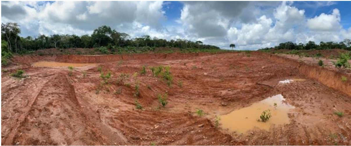
One of the borrow pits
