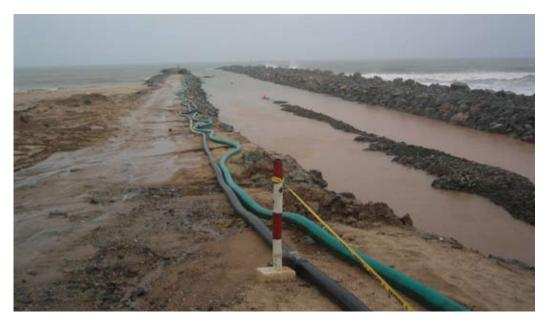
Nigeria: West Africa Gas Pipeline—Embankment protecting the gas pipeline as it reaches the shore of Takoradi in Ghana
